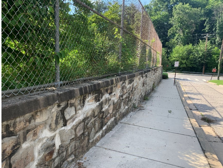
Lot 1 Retaining Wall
