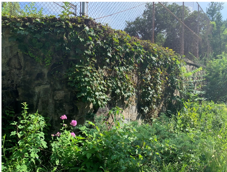
Lot 1 Retaining Wall
