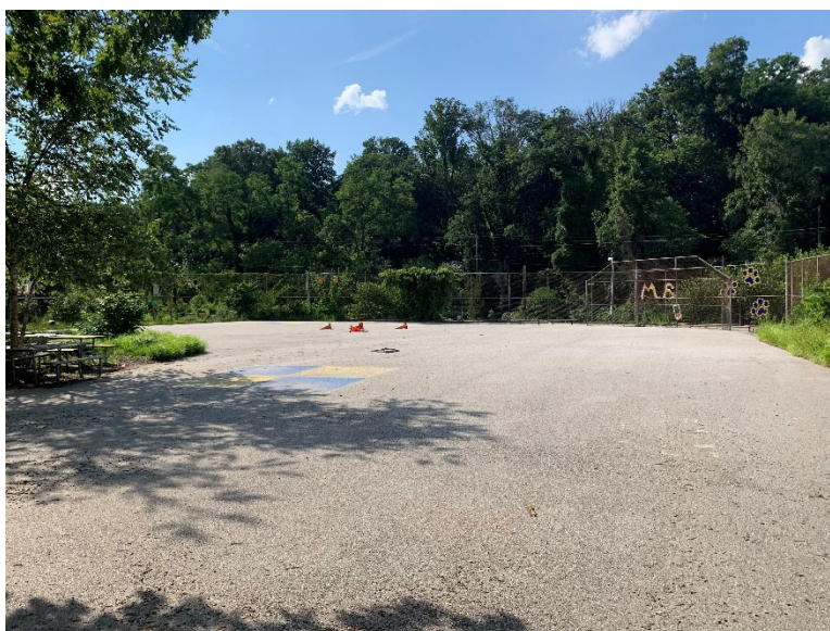
Lot 1 Asphalt Surface
