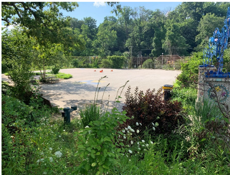
Lot 1 Asphalt Surface
